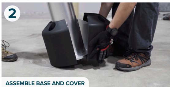
ASSEMBLE BASE AND COVER
